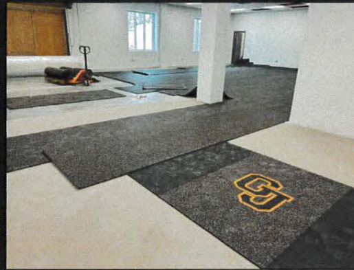
Weight Room Flooring
